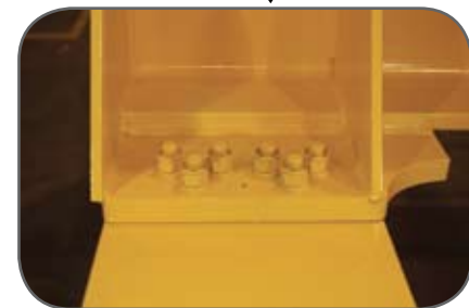
Standard bolted girder connection plates
